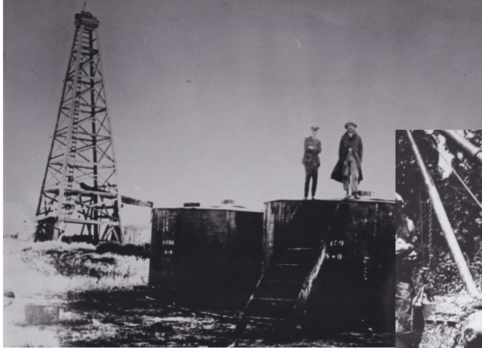
Picture taken in Oklahoma in 1920 showing the gauger using a pole to measure depth of crude oil in the producer's tank. This long unwieldy pole was carried on the side of the gauger's car or buggy.
